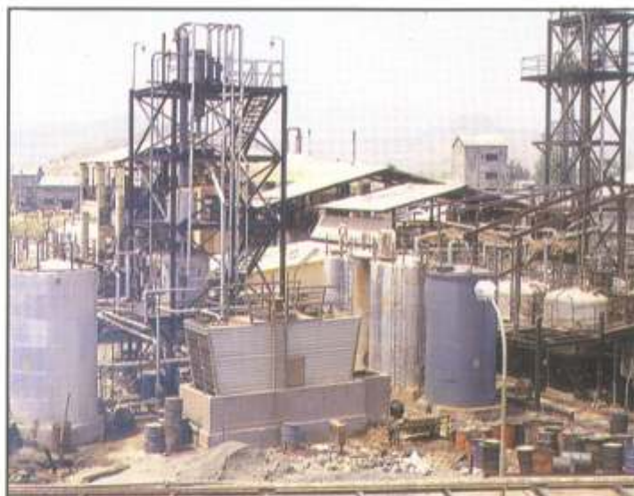
View of the Mahad Plant.
